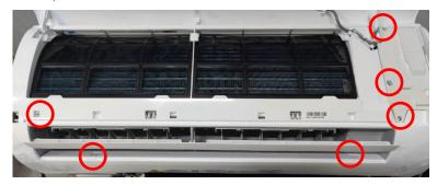
Open the screw cover for the lower screw as shown in the figure, then remove the screw.
